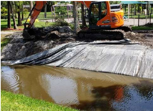
Fig 20. Reference - Embankment stabilization and restoration
