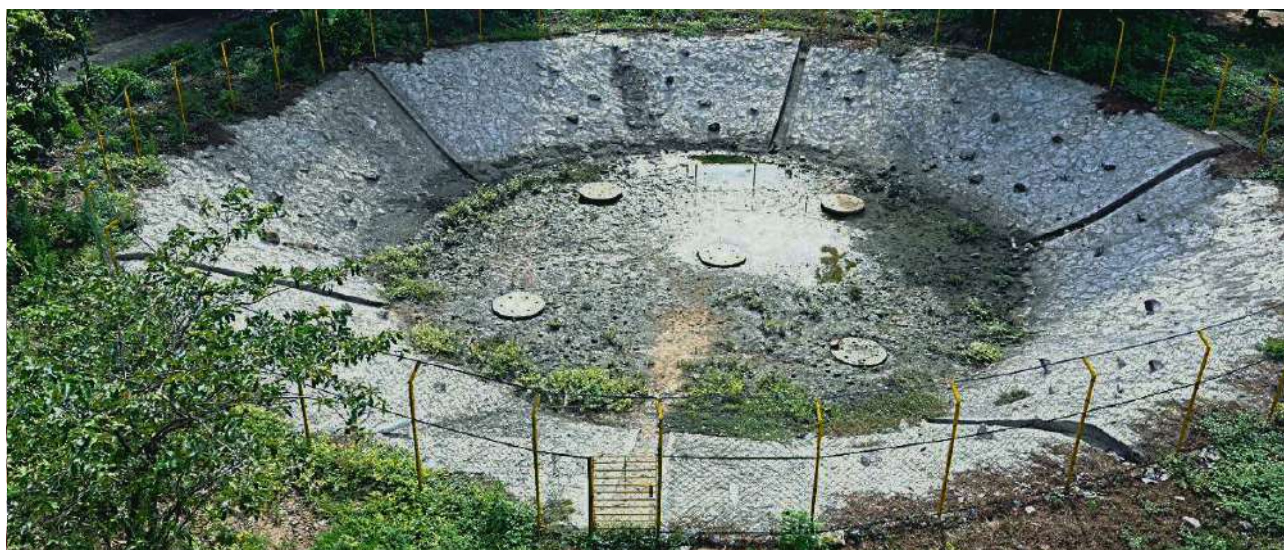
Fig. 10 The sponge park getting ready at Perambur Murasoliman Park with a centralised structure for water harvesting
