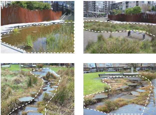
Fig. 2.27 includes permeable paving, raingarden and biofiltration swales
