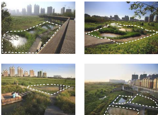
Fig. 2.36 Images of vegetated swales that capture and filter storm water
