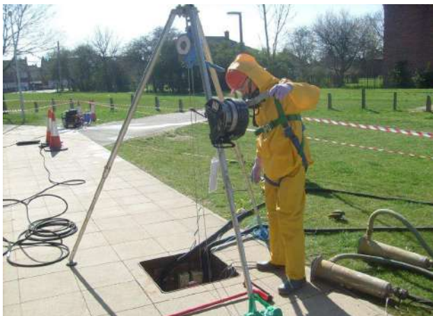
Fig 4.25. Reference - Rainwater harvesting pit cleaning
