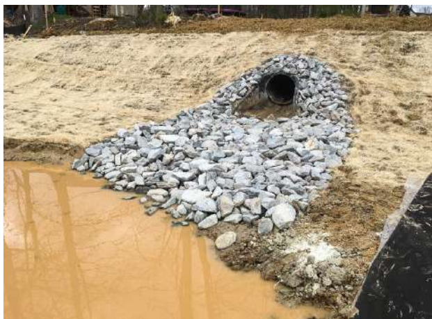
Fig 22. Reference - Energy dissipating inlet channels for ponds
