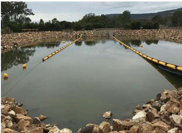
Fig 21. Reference - Pond with baffles
