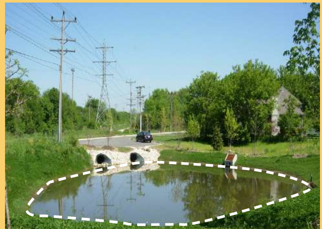
Fig. 2.71. Reference Images of Retention pond
