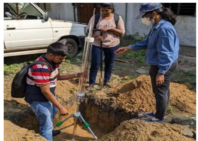
Fig. 2.49 Reference - Infiltration test conducted using
