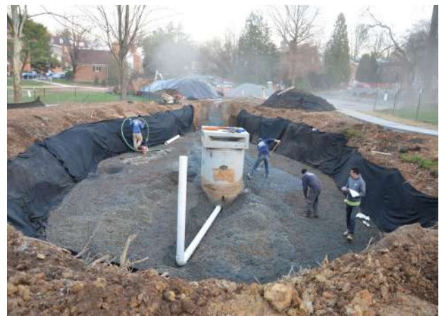
Fig 3.7. Reference - Construction of Bio retention ponds
