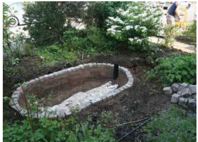
Fig 13. Reference - Rain garden under construction
