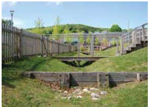
Fig 11. Reference - Timber check dams, Rednock School, Gloucestershire
