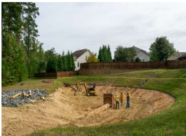
Fig 3.8. Reference - Construction of Infiltration ponds
