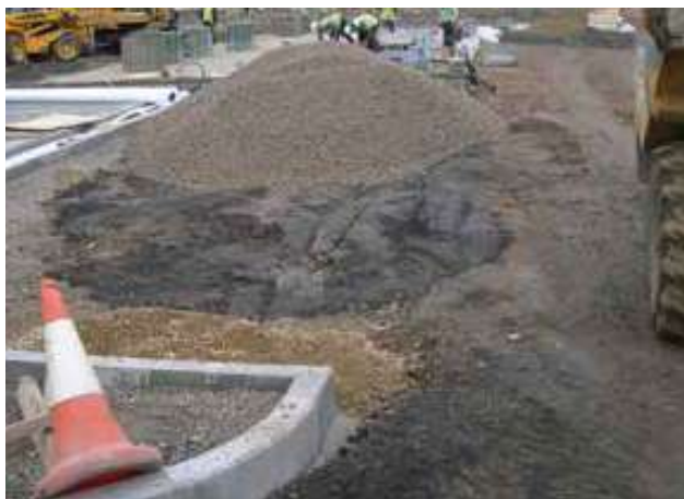
Fig 3.5. compaction of sub-grade below pervious construction intended to infiltrate water
