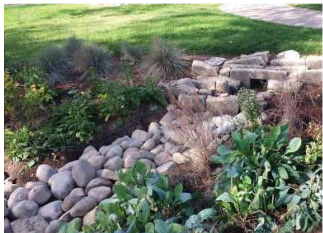
Fig 4.23. Reference - Extension of a velocity dissipator
