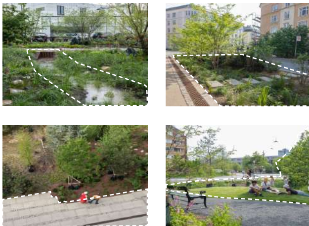
Fig. 2.18 Various sustainable drainage systems
