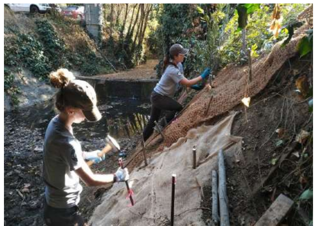
Fig 3.11. Reference - Bioengineering of the soil
