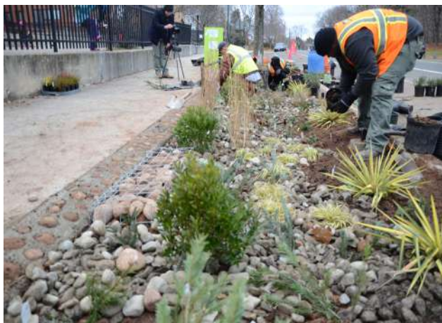
Fig 3.6. Reference - Construction of Bioswales
