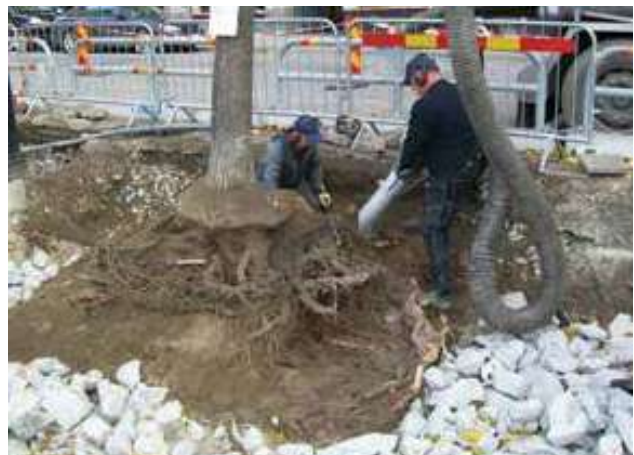
Fig 27. Reference - The use of structural growing media in retrofitting
