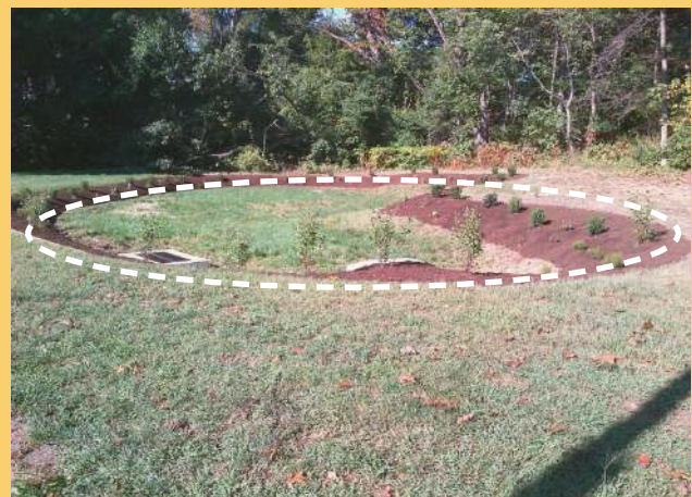
Fig. 2.74. Reference Images of Infiltration Basin
